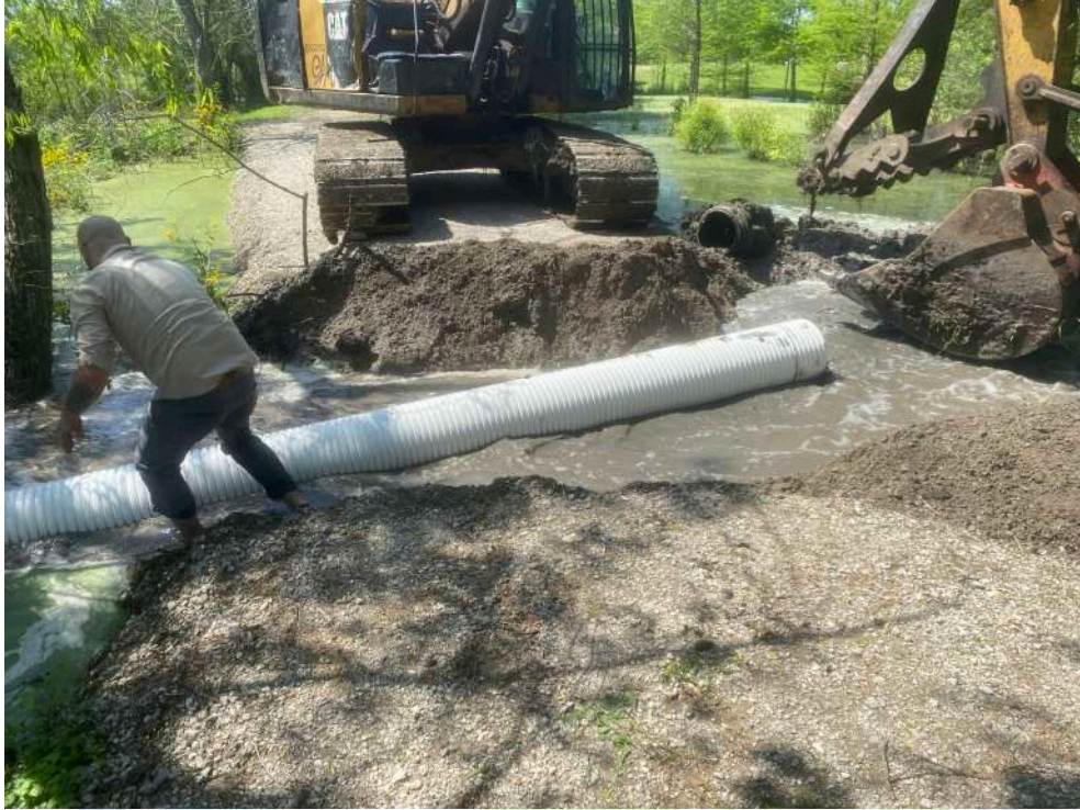
Devin Theobald getting wet while positioning the culvert.
